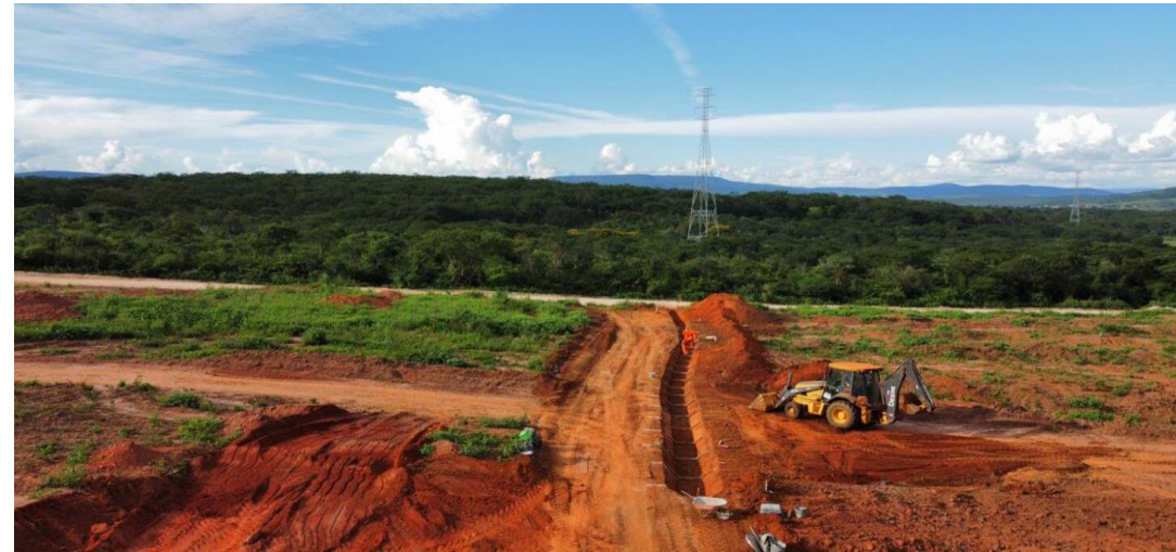
Construction at Sigma Lithium Grota do Cirilo project
