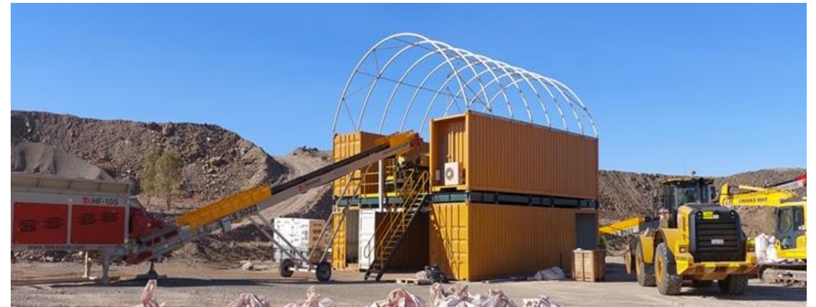
Mechanical Sorting Plant Setup at Nullagine, WA
