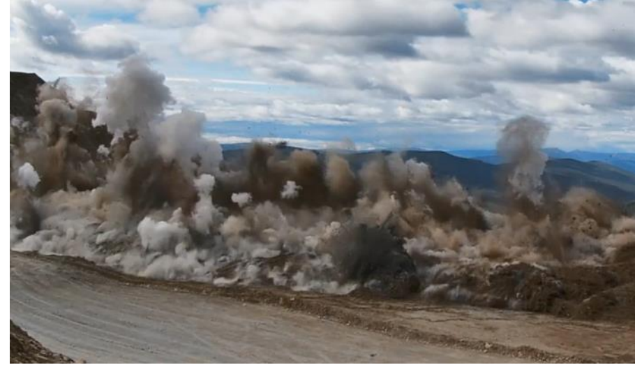
Blasting in Eagle Phase 1
