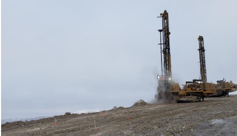
Drilling in Eagle Phase 2
