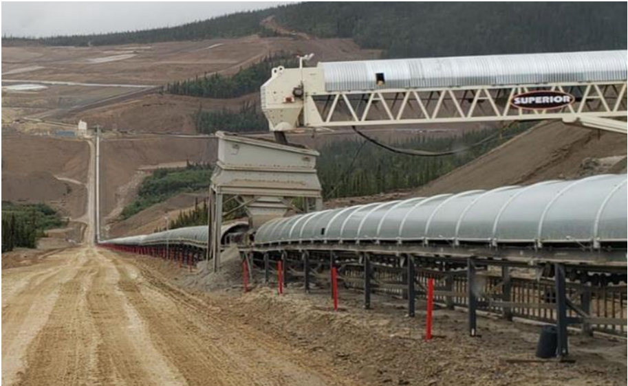
Overland Conveyor Linking Secondary to HLF
