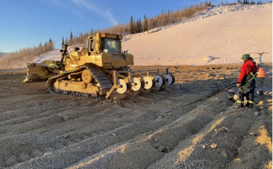
Installing Drip Emitters with CAT D6 Dozer
