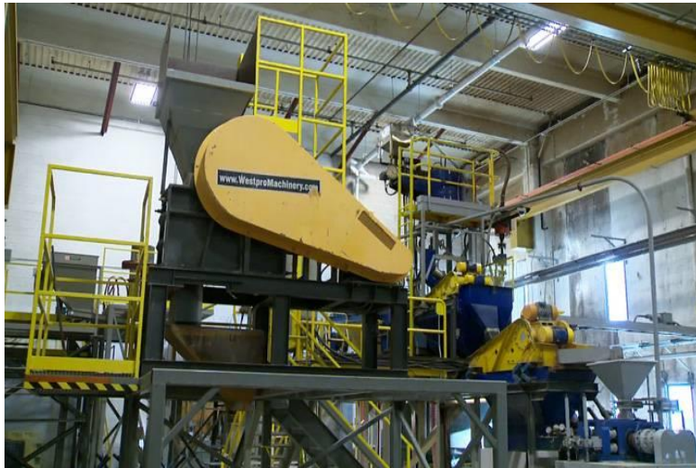
Pilot Processing Plant (1,000 tonnes per annum capacity)
