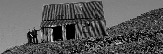
SOLO MINE CABIN
