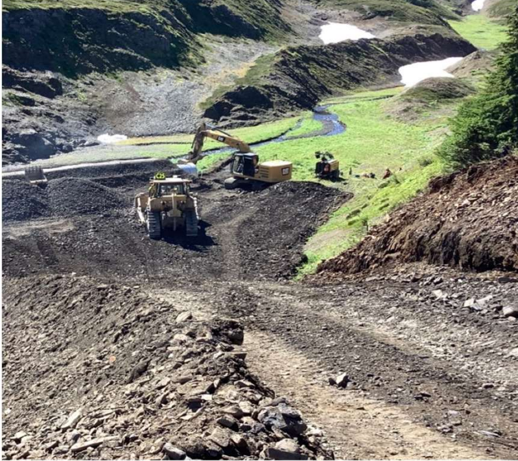
Coulter Creek Access Road
