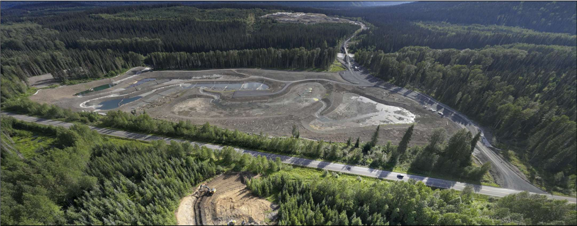
Glacier Creek Fish Habitat Construction Completed
