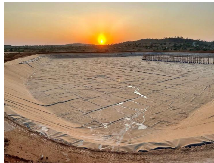
Figure 3. Liner installation at TSF 2.2
