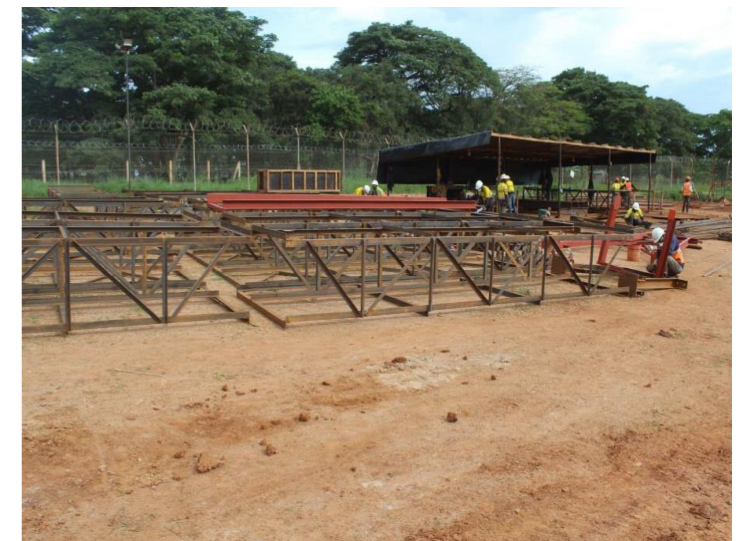
Figure 4. Fabrication of beams for the new crushing circuit
