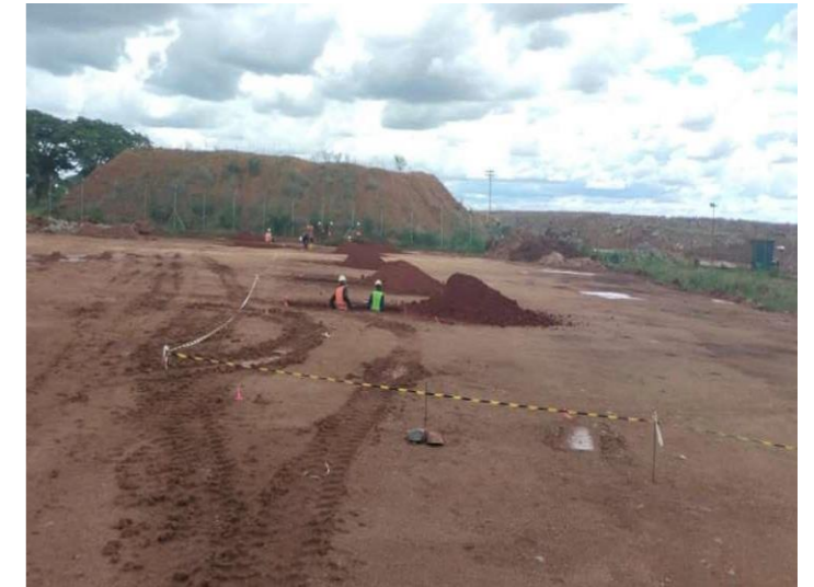
Figure 2. Excavation work & planning of future milling site
