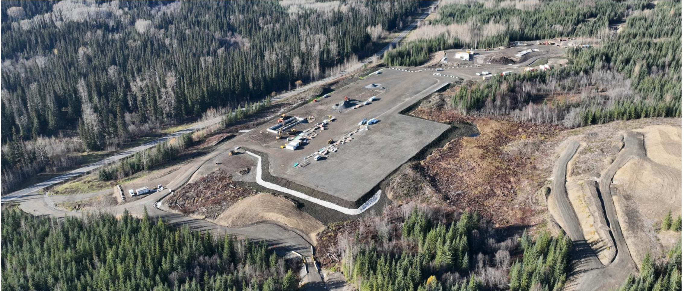
BC Hydro's Treaty Creek Terminal
