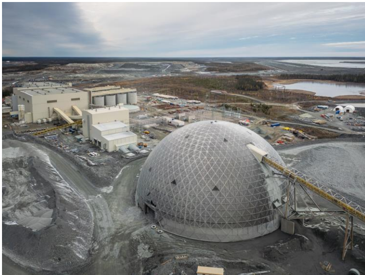
Detour Lake operations
