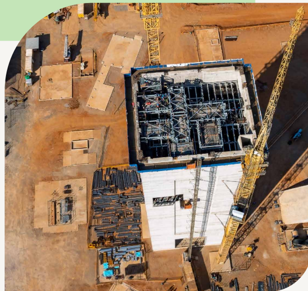
Base of Shaft 2 headframe under construction
